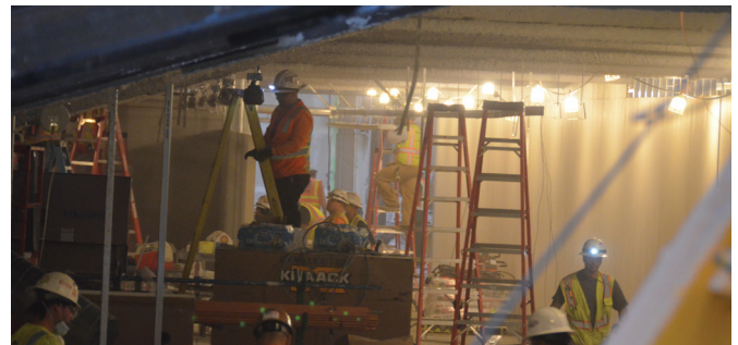
Nearly 90 percent of TBIT's construction workforce live in Southern California
