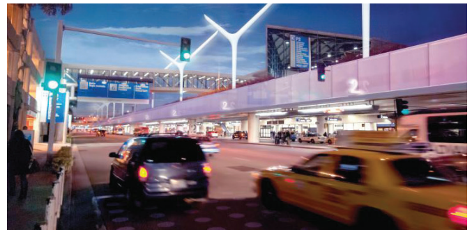
The sculptural LED light poles and light band will improve lighting as well as assist pedestrians and motorists in navigating the LAX Central Terminal Area.
